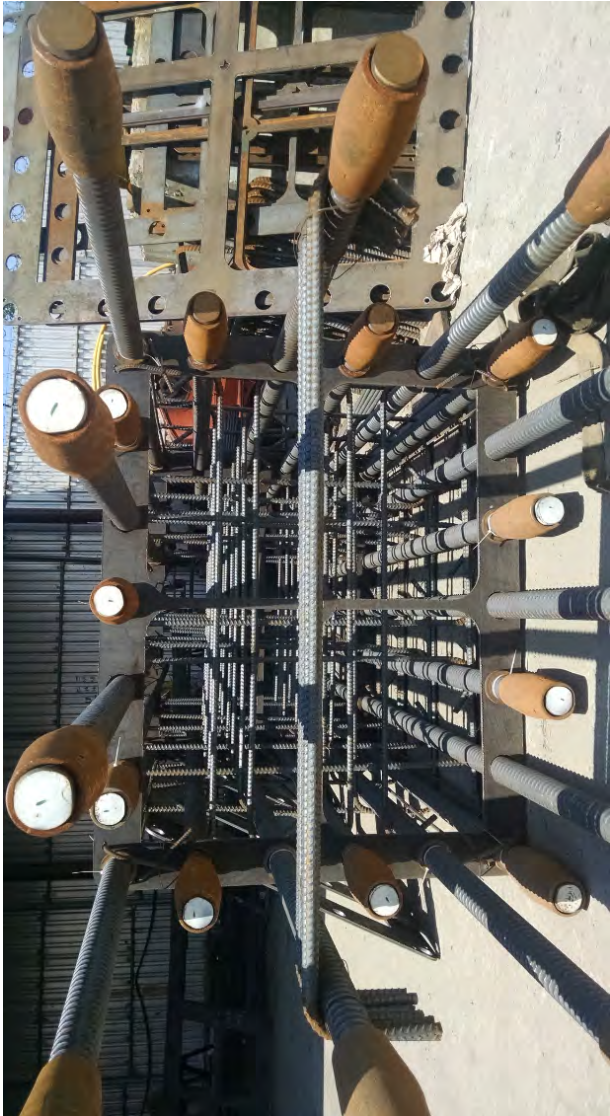
ABOVE: 99 HUDSON STREET, NEW JERSEY. CAGES FABRICATED USING #20 GRADE 80 SSI THREADED BAR.
