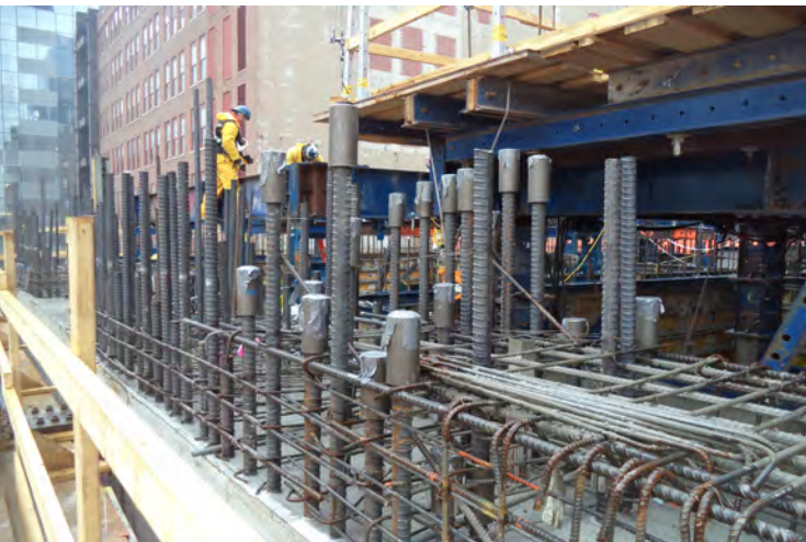
LEFT: STICK UP LENGTHS AFTER CONCRETE SLAB HAS BEEN POURED
