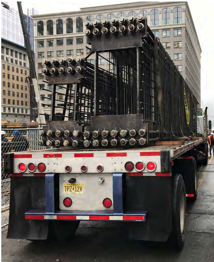
ABOVE: LINK BEAMS COMPLETELY PREFABRICATED WITH HARDWARE AND LATERAL REINFORCEMENT PRIOR TO SHIPPING TO SITE.
