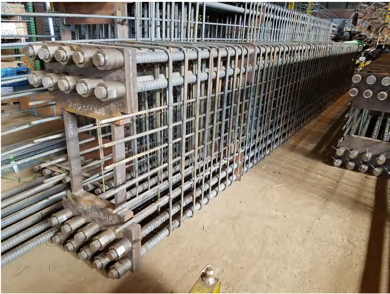
ABOVE: PREFABRICATED LINK BEAM, WITH HARDWARE AND LATERAL REINFORCEMENT PRIOR TO SHIPPING TO SITE
