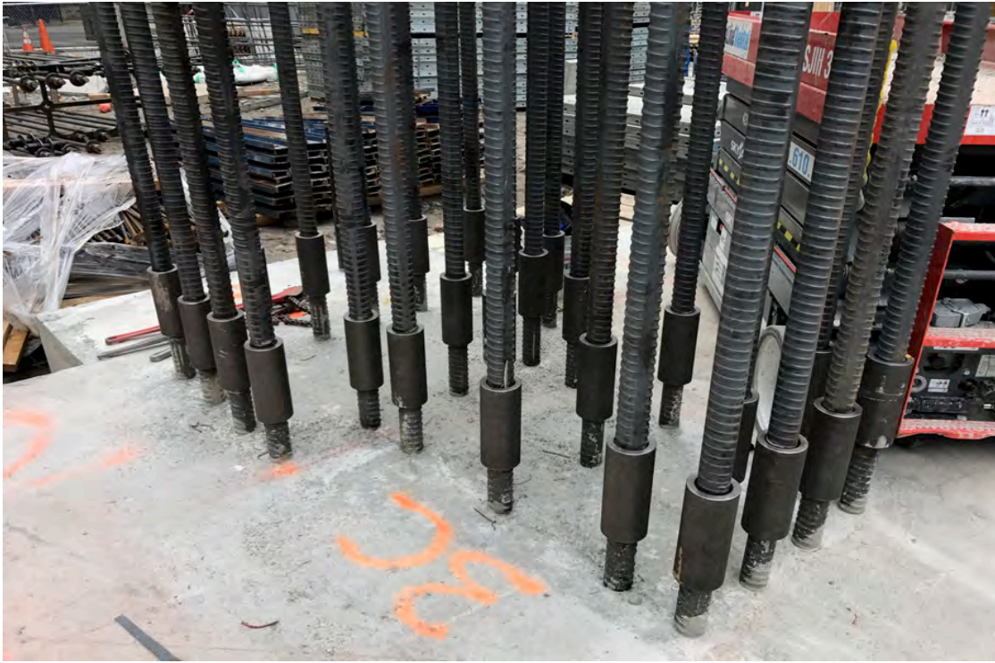
ABOVE: 99 HUDSON STREET, NEW JERSEY. CAGES FABRICATED USING #20 GRADE 80 SSI THREADED BAR.
